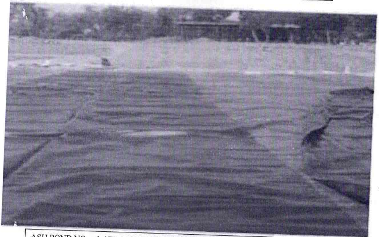
ASH POND NO. - 1 AFTER PUTTING UP THE HDPE LINING (PHOTOGRAPH - 8)
