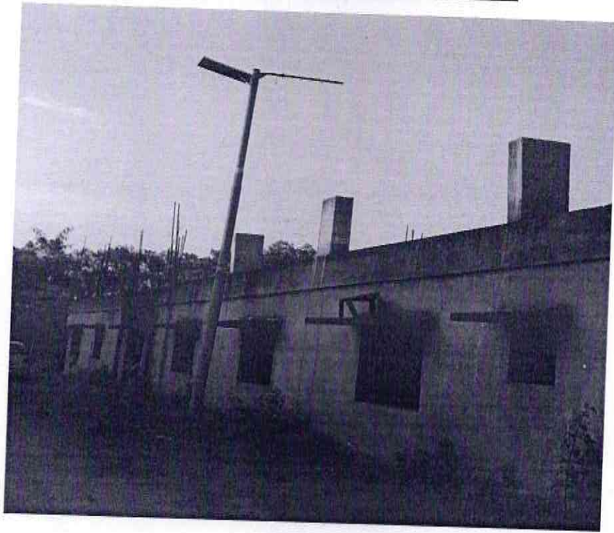
Solar Light Mounted in Street light Pole
